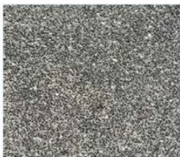
Parking Concrete, Black Ox., Exp. Aggr. Poured in Place
